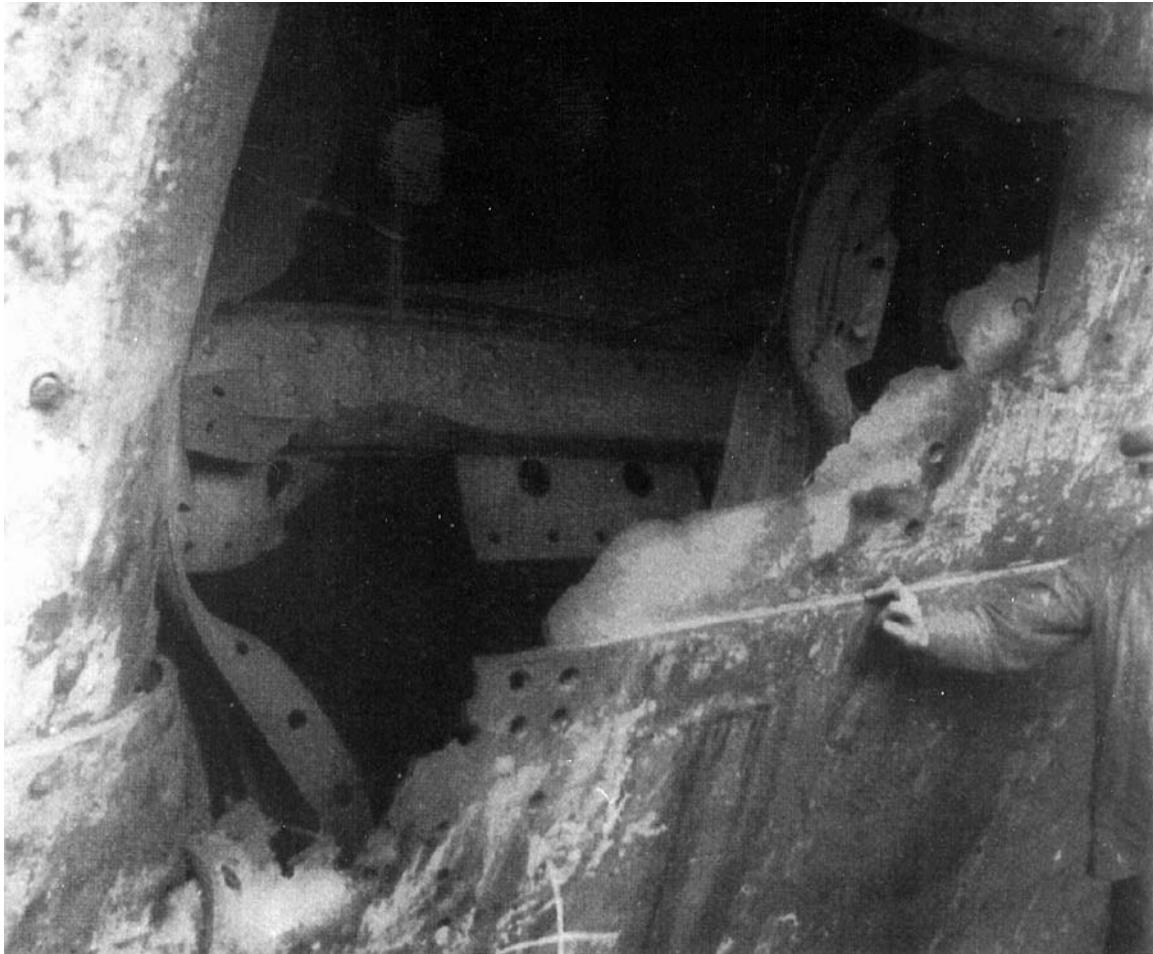
Figure 6: A close-up of the damage to the RMS Olympic due to collision with the HMS Hawke in the Solent in 1911. Note the man for scale. A considerable amount of plasticity in the hull plates is indicated by the bending and twisting seen in the picture. Note missing rivets. Photo from [25].
